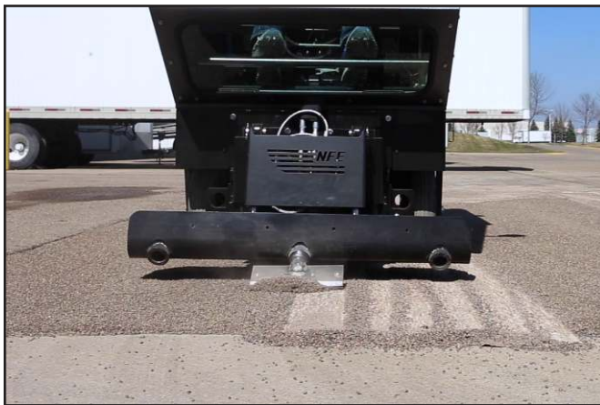
Machine scraping epoxy-covered concrete.
