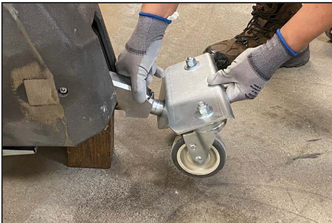
Installing transport wheels.
